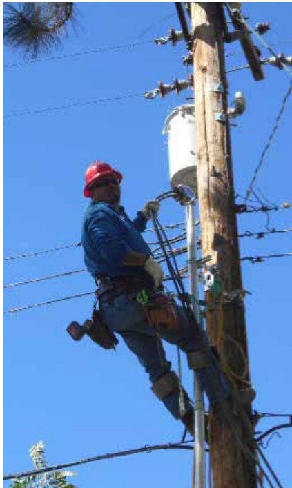
Electric Lineman undertaking system upgrades on the electric distribution system.
