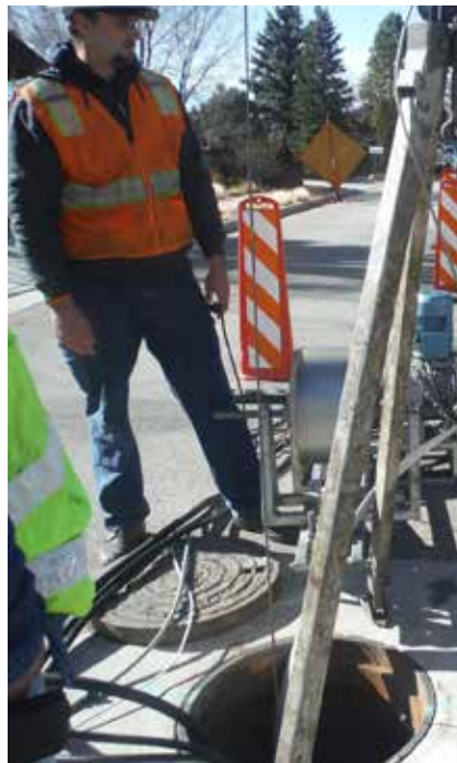
Trenchless replacement and rehabilitation of sanitary wastewater collection pipes.
