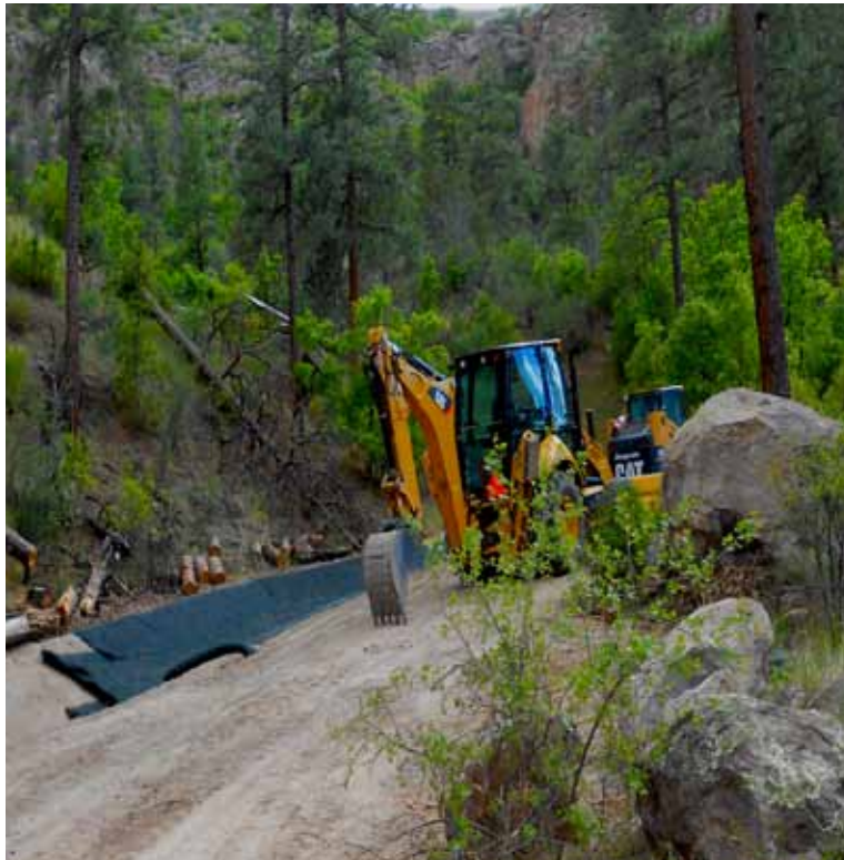
Contractor installs a roadside bar ditch on the access road to Los Alamos Reservoir.
