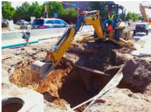
New sewer line being installed on Central Avenue in coordination with Public Works' Central Road Improvement project.
