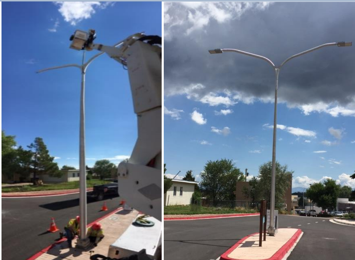
Traffic Crews installed a new double arm light pole at 40 th Street and University on August 23 rd .
