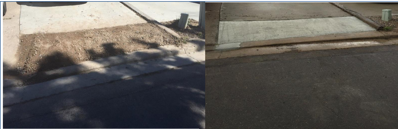
Before and after images at 1312 Sage. There was a utility line break, Streets Crews repaired the drive pad at the entrance.
