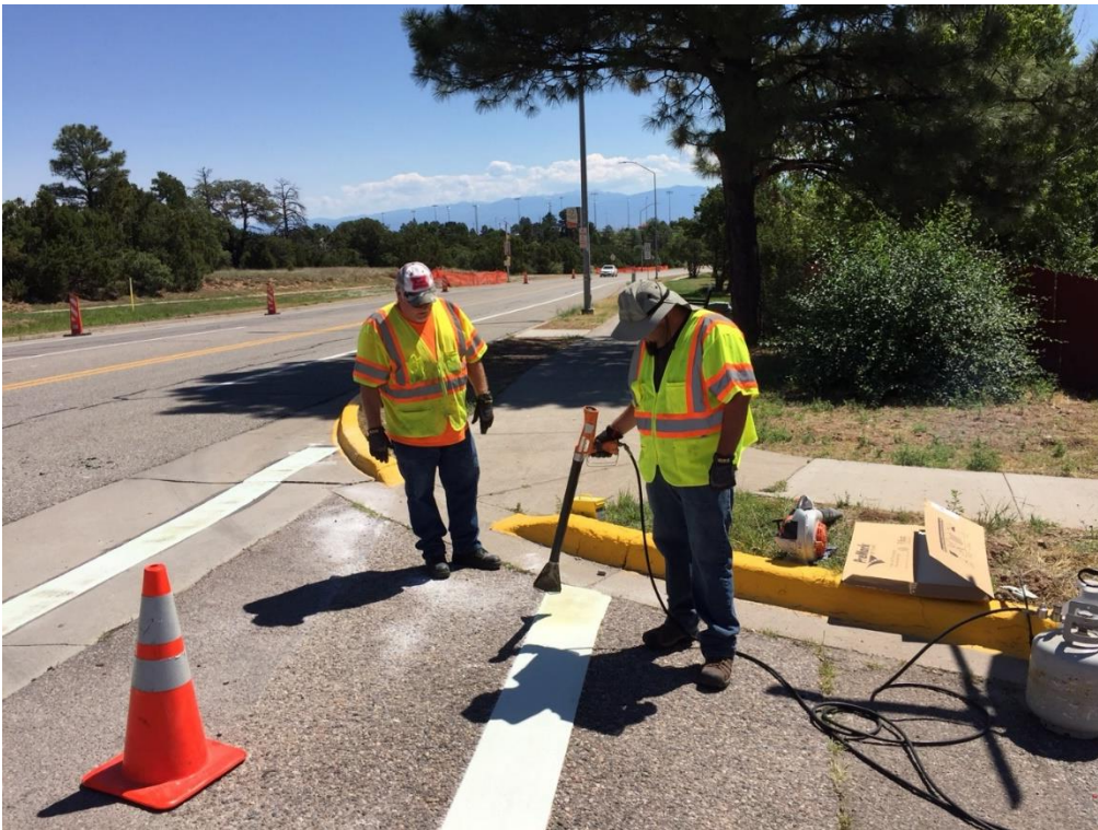
Traffic Crews eradicating and replacing crosswalks throughout the County.
