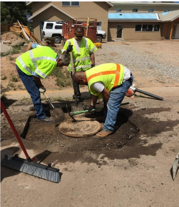
Crews work on manhole repairs for the Department of Public Utilities.
