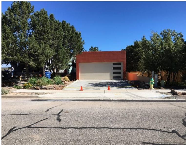
Street crews removed and replaced a drive pad at a 25% slope to a 7% slope.
