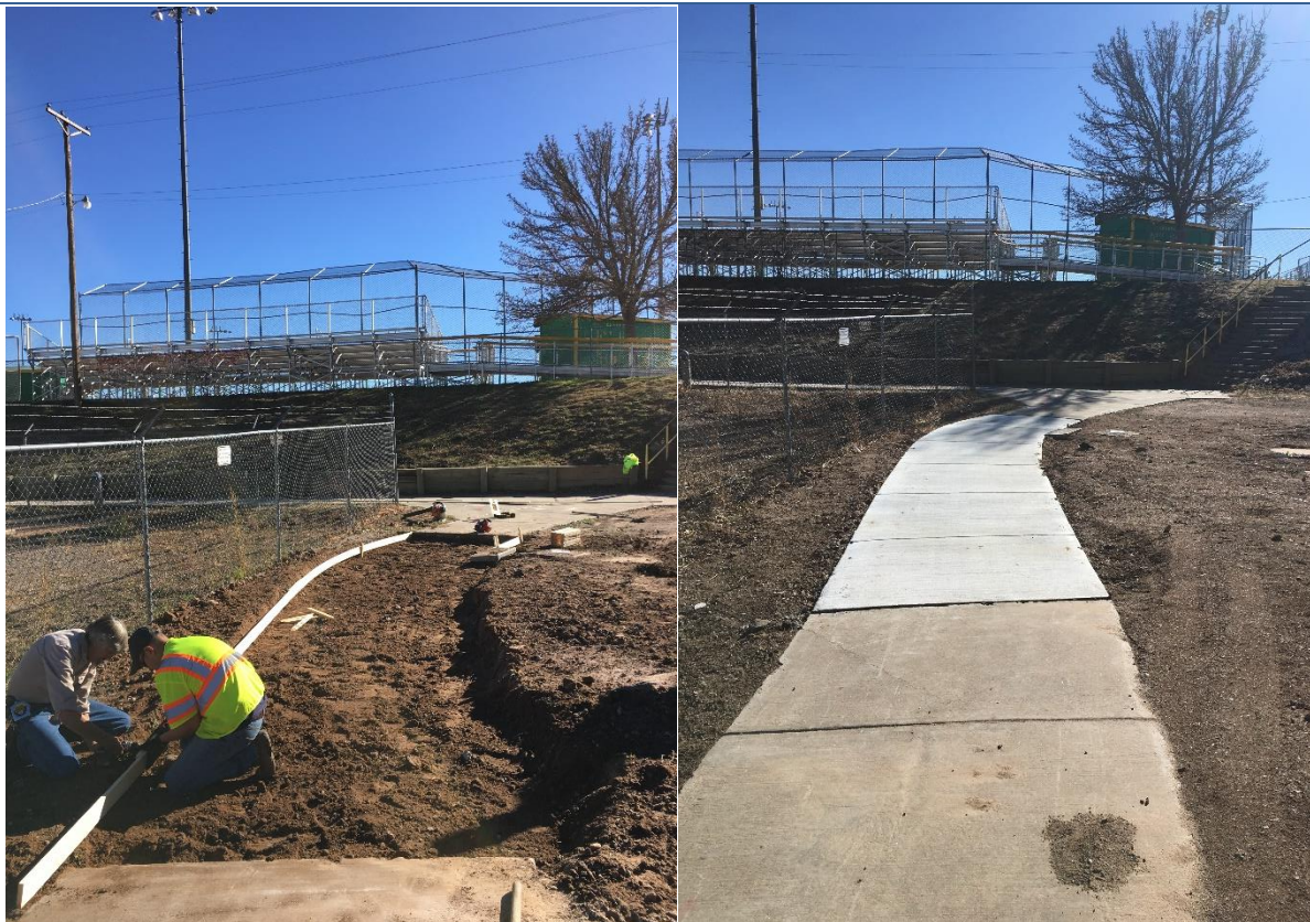
Crews are replacing a section of sidewalk at North Mesa due to a water main break.
