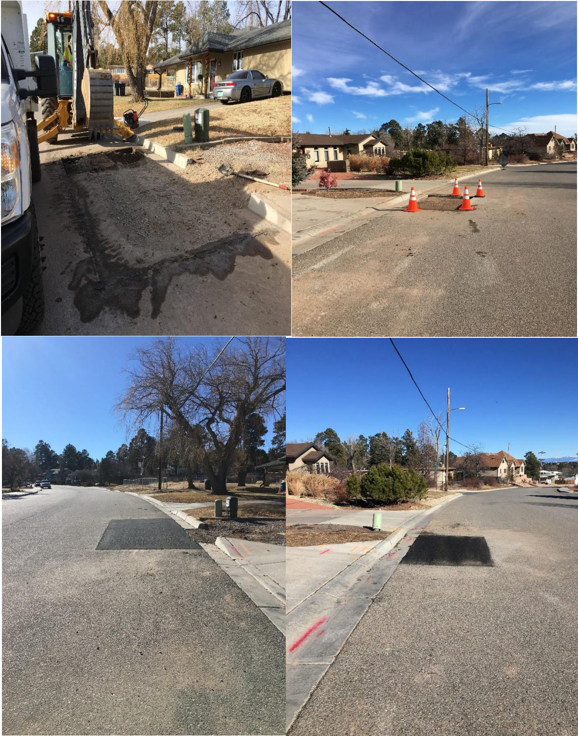
Crews repaired and patched two utility water breaks at Sandia and Trinity Loop
