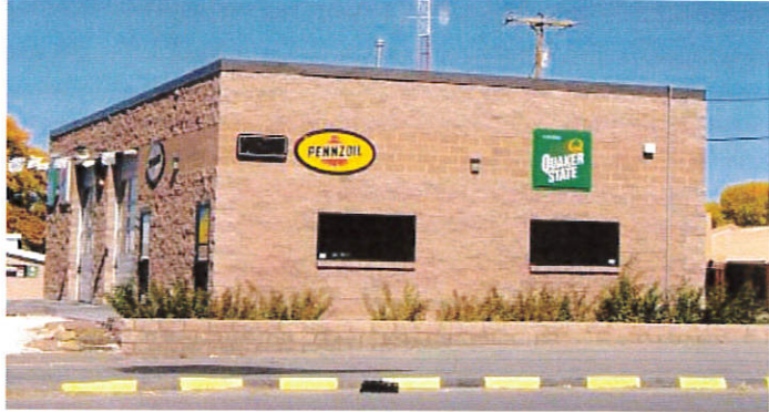
Illustration 1. This simple box-shaped building does not meet the requirement for complex massing. (It also fails to meet the ordinance requirement for exterior materials since it is composed entirely of concrete block.)
