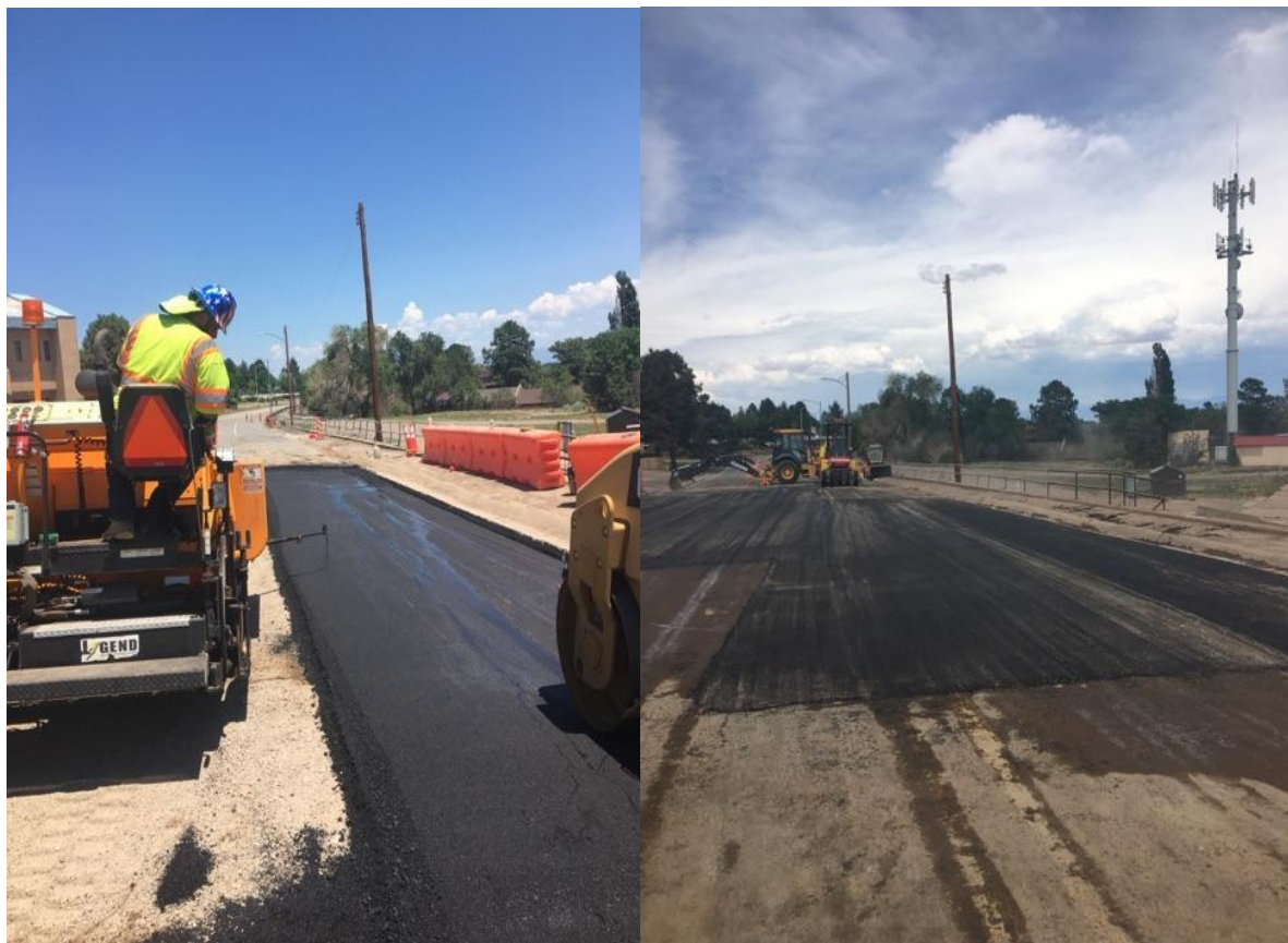
Crew members assist Utilities GWS on Trinity Drive between DP Road and 4 th Street where a sinkhole formed due to a leaking sewer main.
