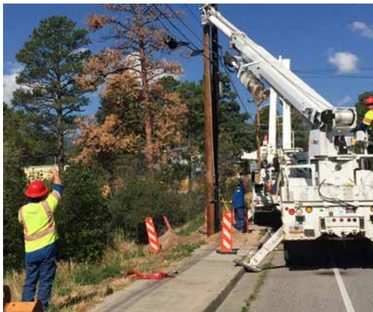
DPU's electric linemen upgrade the overhead electric system.
