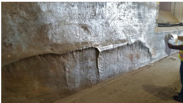
Existing buckled steel.
