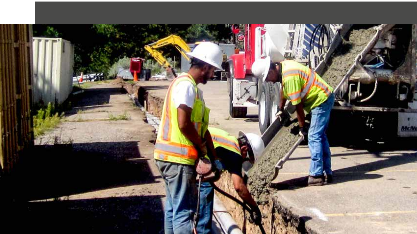
Electric primary lines are installed for the new Los Alamos Switchgear Substation by the hospital.
