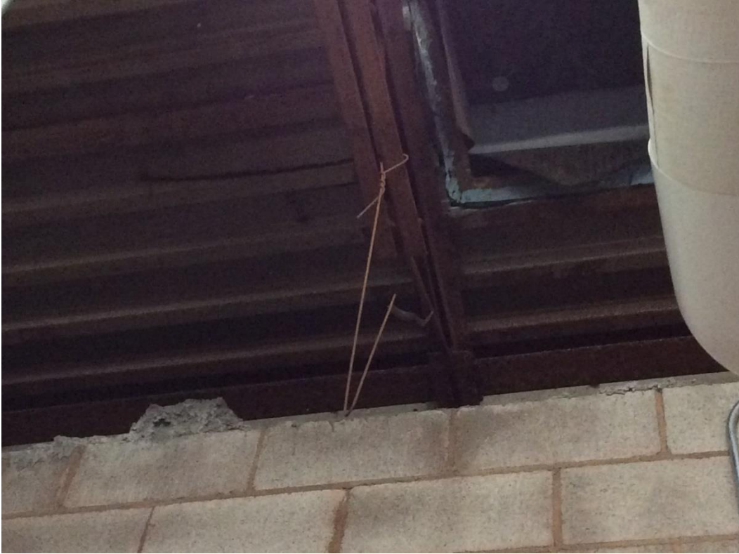
Figure 5 – Mechanical Room Roof Beam Corrosion
