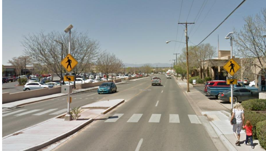
Rectangular Rapid Flashing Beacons (RRFB's)
