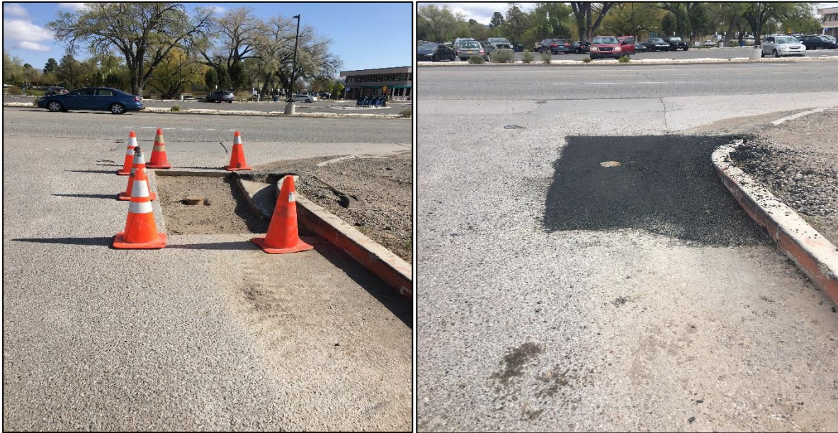
Crews repaired a section of asphalt that had to be removed for Utilities to repair a line at 2101 Trinity Drive.
