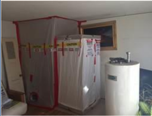
Home Rehabilitation Project (Los Alamos) Boiler Replacement and Asbestos Removal
