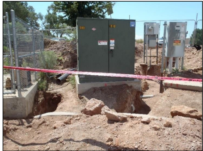
Utility yard trenching for new gas/electric
