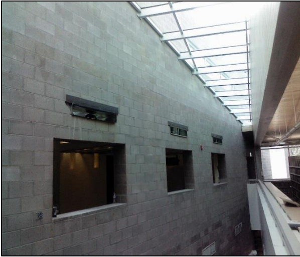
New return air penetration (smaller holes)
