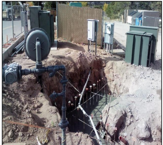
New gas meter and transformer (upper)
