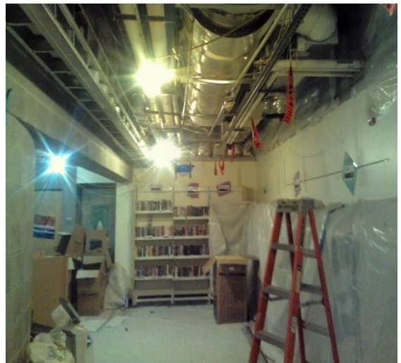
New air intake structure
