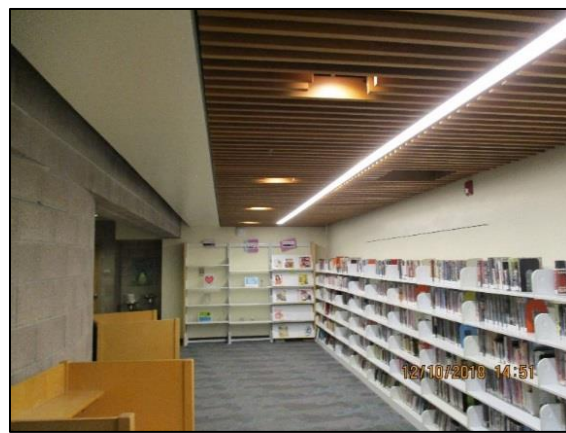
Newly installed wood ceiling and LED lighting in lower level.
