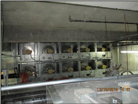
Newly installed fan units.
