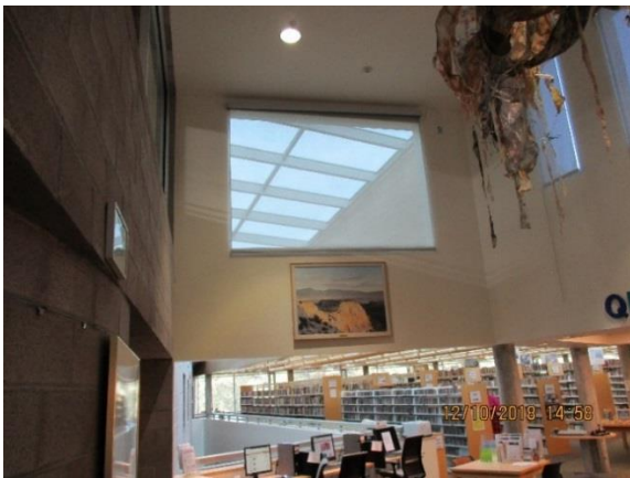
Newly installed sun blocking screen
