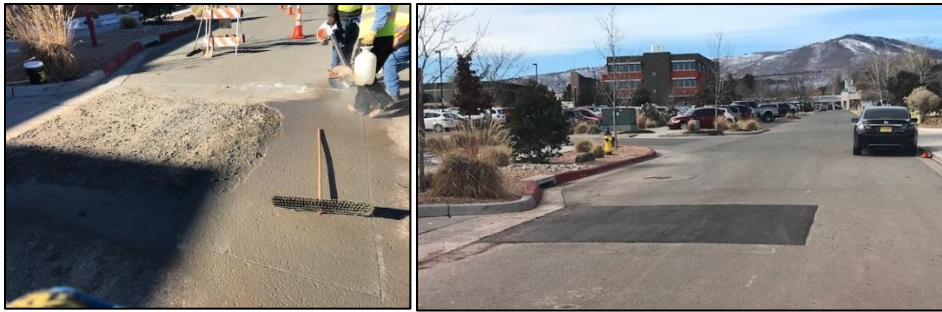
A repair on Iris Street near the municipal building after DPU crews repaired a gas leak.
