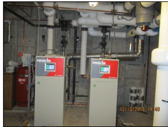
Newly installed boilers.
