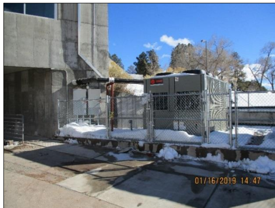
Chiller Units and new piping
