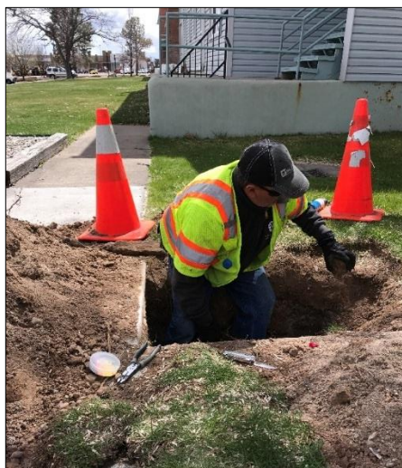
Traffic Electricians tracked down and repaired faulty wiring at 6th and Iris.
