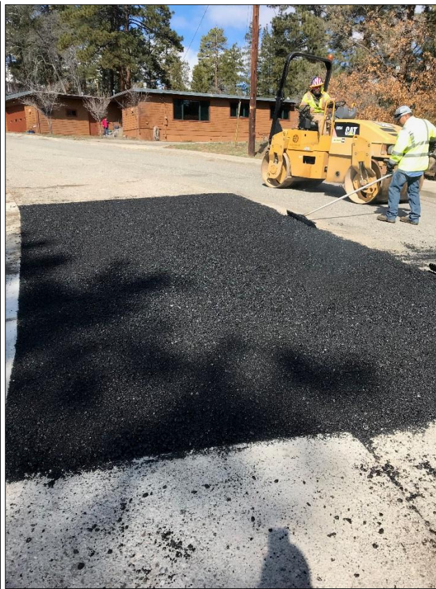
Crews have been patching sections of asphalt on 33 rd and 34 th Street.
