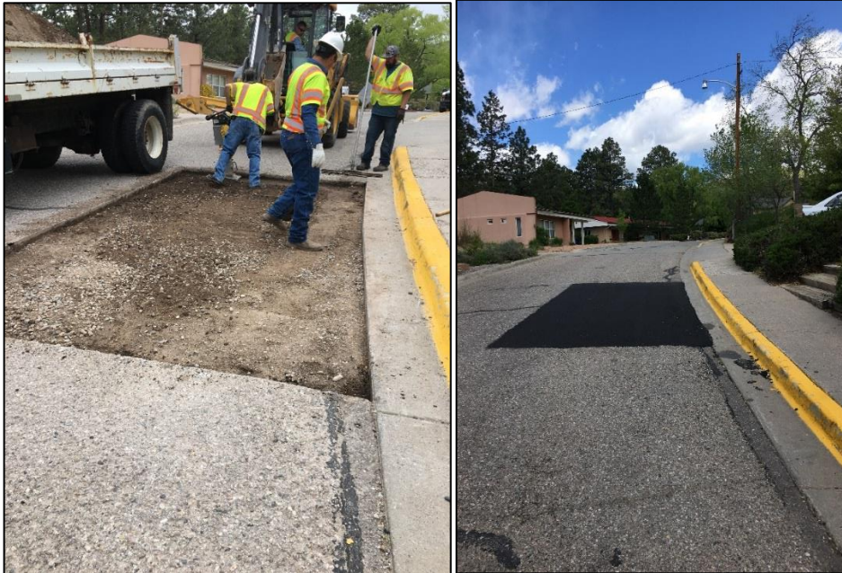
Crews are seen repairing a section of road on Fairway Dr. where utilities made a cut to repair a line.
