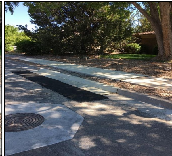
Crews repaired curb and gutter and sidewalk at 718 Jeffrey Pl. due to a water break.
