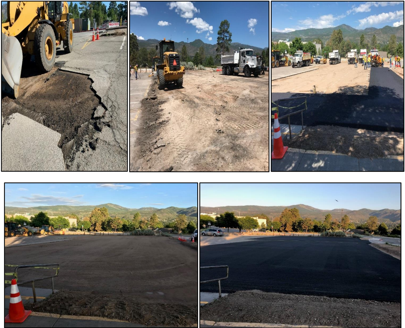
Crews removed existing asphalt that failed at the Mesa Public Library and laid new asphalt.
