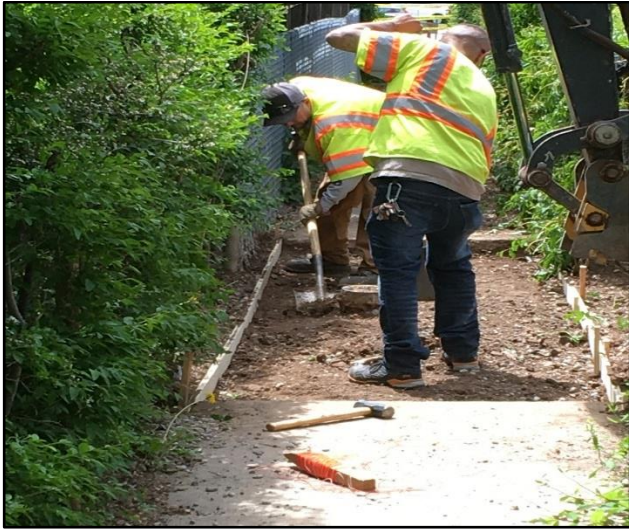
Crews repaired a section of sidewalk at 11th St. due to a water break.
