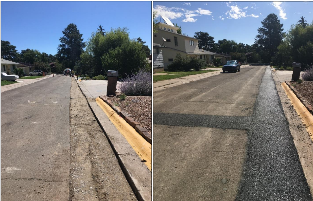
Crews started repairing shoulders along Ski Hill Road. This work is being done as a preservation effort to stop the existing shoulders from continuing to unravel.
