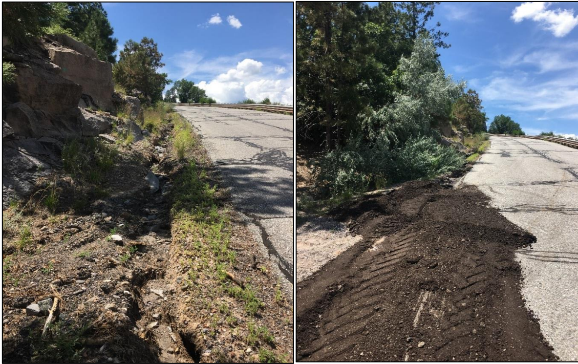
Crews started repairing shoulders along Ski Hill Road. This work is being done as a preservation effort to stop the existing shoulders from continuing to unravel.
