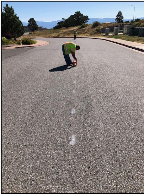
Crews striped a new double yellow line and installed a 25 MPH sign on Entrada Dr.
