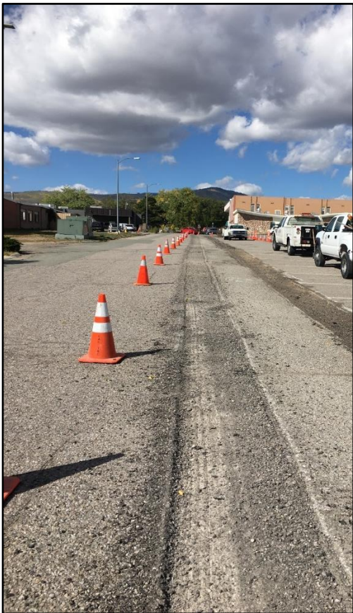
Crew repaired several sections of broken asphalt along Deacon Street.
