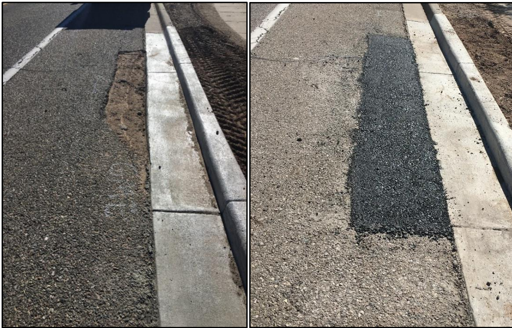
Crews patched a section of asphalt on San Ildefonso Road
