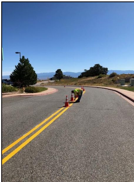
Crews striped a new double yellow line and installed a 25 MPH sign on Entrada Dr.
