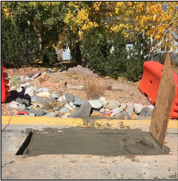
Crews repaired the sink hole and placed an asphalt patch.
