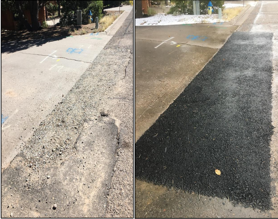
Before and after images of asphalt patch work done as part of Traffic and Streets division assisting Utilities with a water main break on Totavi.
