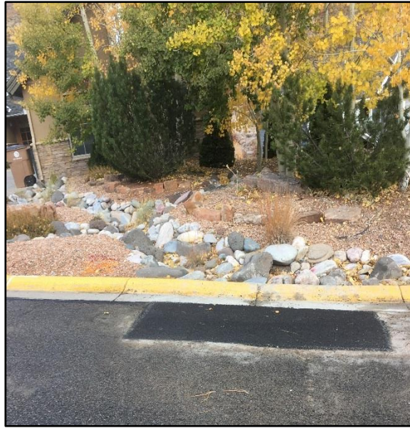
Crews repaired the sink hole and placed an asphalt patch.
