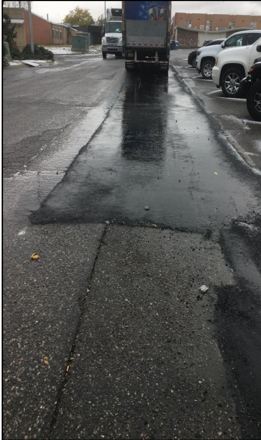
Crew repaired several sections of broken asphalt along Deacon Street.
