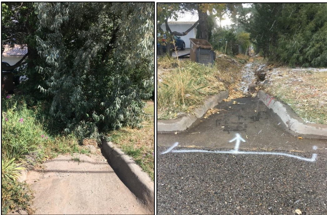
Crews cleared tree limbs and brush from a drainage ditch on Loma de Escolar.
