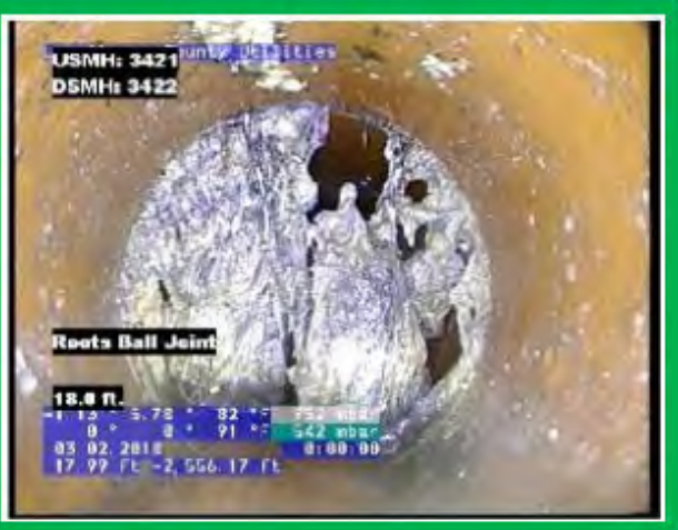
Sewer Video of Root Blockage
