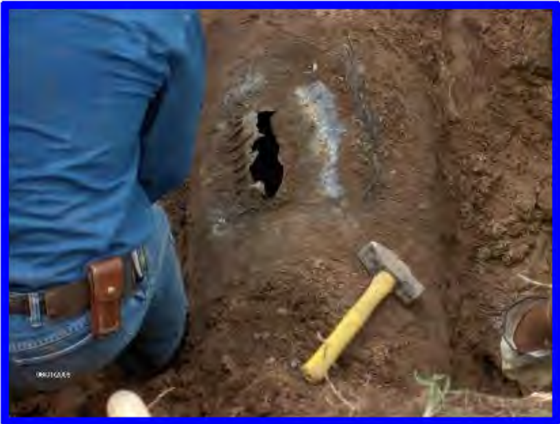
Leak in Concrete Cylinder Pipe
