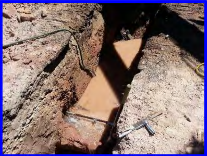
Service Line Leak with Multiple Repair Clamps
