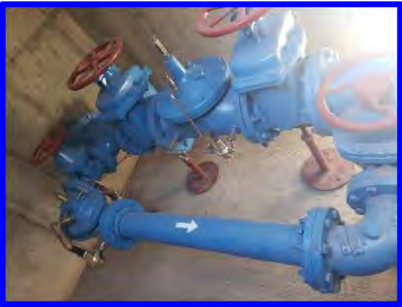
Water Pressure Reducing Valves Refurbishment (Left Before & Right After)
