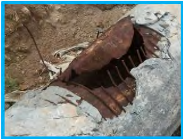
Concrete Cylinder Transmission Line Failure
