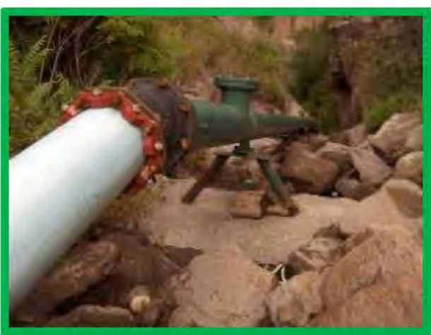
Above Ground and Inaccessible Sewer in Canyon
