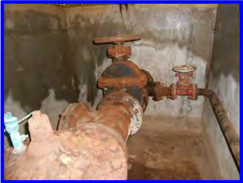
Water Pressure Reducing Valves Refurbishment (Left Before & Right After)
