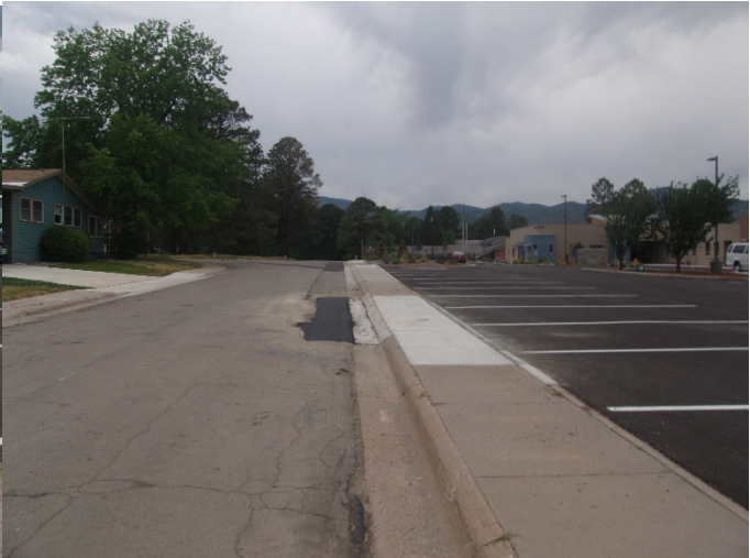
Repaired and replaced curb, gutter, and sidewalk at 1400 Sage due to a utility break.
