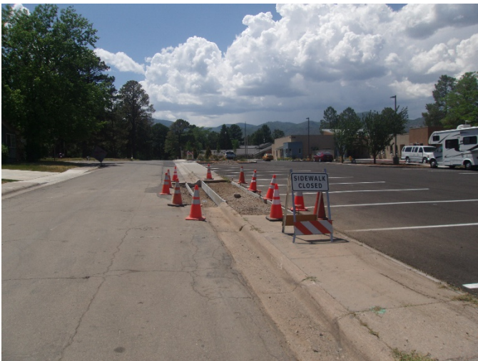
Repaired and replaced curb, gutter, and sidewalk at 1400 Sage due to a utility break.
