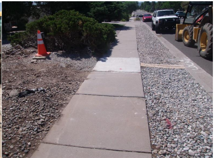
Repaired and placed a sidewalk stone on Meadow Lane that a resident damaged when he pulled out shrubs with a wrecker.
