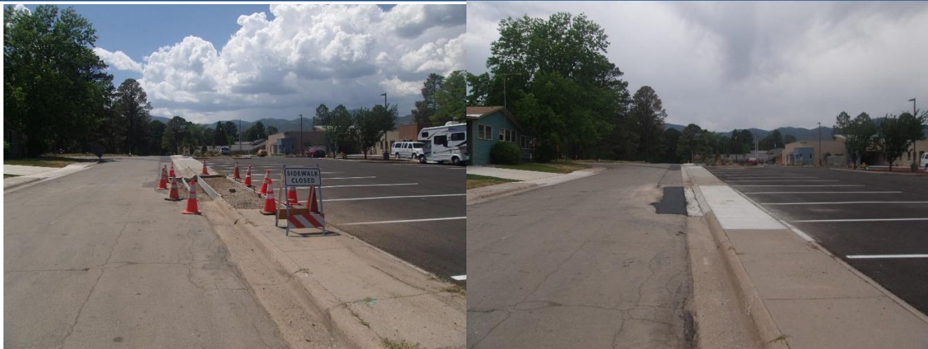
Repaired and replaced curb, gutter, and sidewalk at 1400 Sage due to a utility break.
