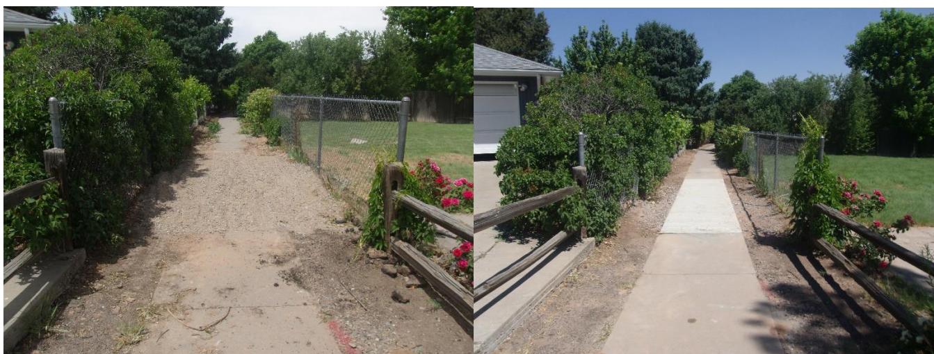
Crews repaired, replaced, and dressed back the sidewalk that was removed on Jeffrey Lane due to a water break.
