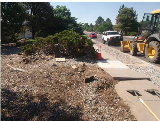
Repaired and placed a sidewalk stone on Meadow Lane that a resident damaged when he pulled out shrubs with a wrecker.
