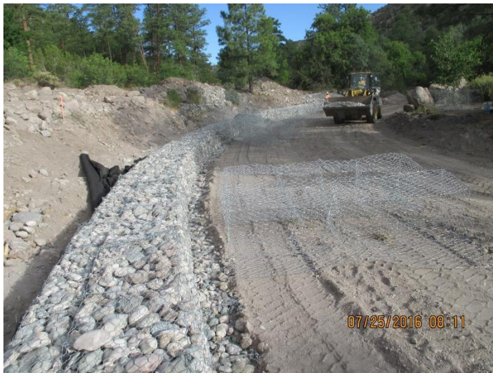
Placement of gabions along roadway.
