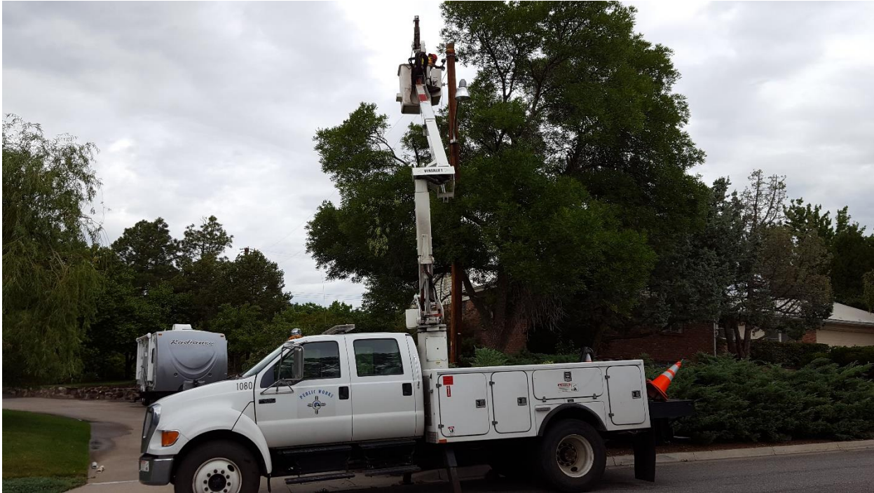
Traffic Crews remove sag from overhead conductors at 277 Andanada. Crews trimmed the trees and moved the wiring.
