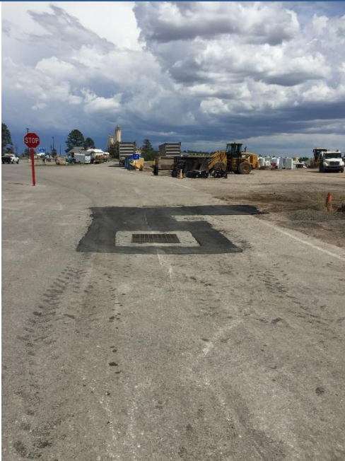
Streets Crews repaired a patch of failing asphalt around a drain at the Eco Station.
