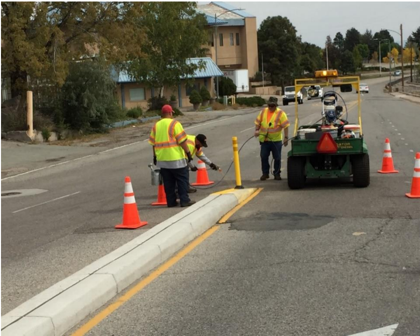
Signs and markings crew have been painting island tips around Los Alamos for better visibility of the islands in the center of the roadway.
