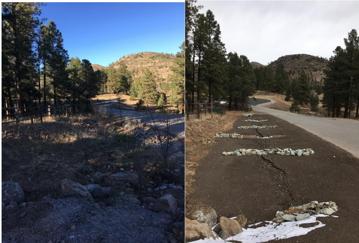
Crews cleaned and built a new drainage ditch at Range Road.
