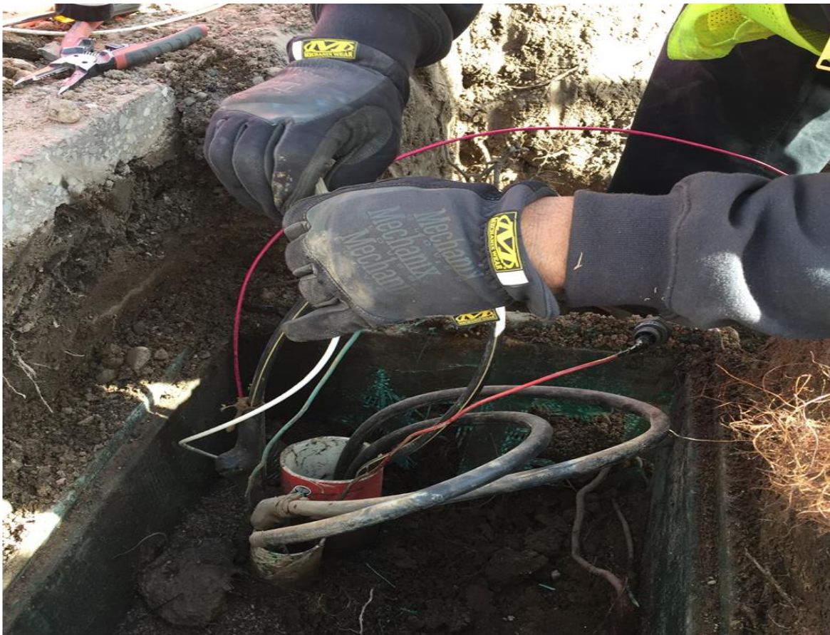
Crews locate a buried pull box to repair a faulted streetlight feed.
