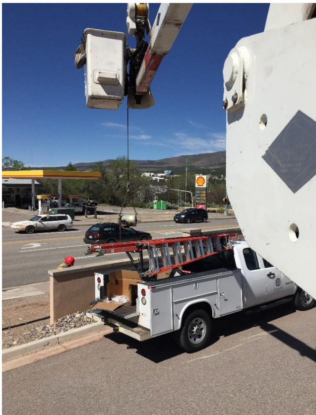
Traffic electricians assisted facilities by lifting a motor to the roof of the Judicial Center.
