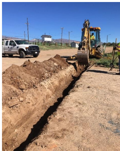
Prep work for the installation of pipe for drainage at the rodeo arena parking area.
