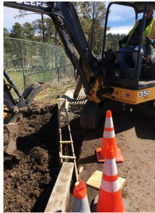
Crew members removed a 6 inch PVC drainage pipe that was plugged and installed a new 12 inch culvert and modified the drop inlet to take more water near the 10th hole T-box at the Golf Course
