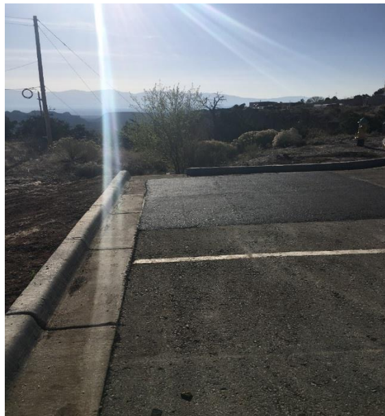
A section of pavement at the Pajarito Cliffs Site collapsed from drainage issues. Staff repaired this section of pavement and fixed any potential for further drainage issues.
