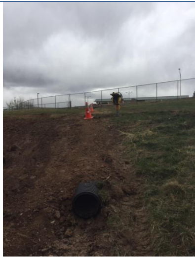
Crew members removed a 6 inch PVC drainage pipe that was plugged and installed a new 12 inch culvert and modified the drop inlet to take more water near the 10th hole T-box at the Golf Course
