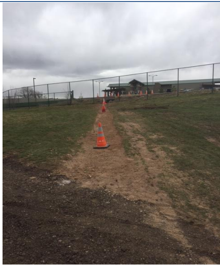
Crew members removed a 6 inch PVC drainage pipe that was plugged and installed a new 12 inch culvert and modified the drop inlet to take more water near the 10th hole T-box at the Golf Course
