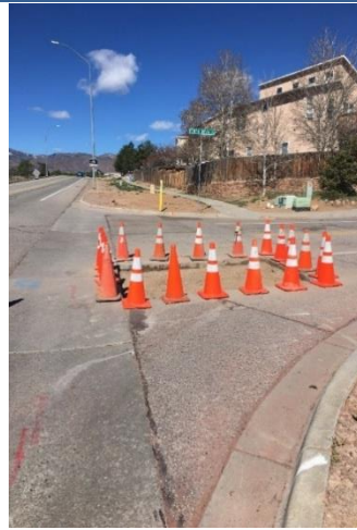
Crew members repaired a section of pavement where a utility line break occurred at North Mesa and San Ildefonso Road.
