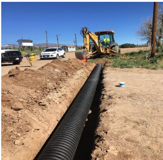
Prep work for the installation of pipe for drainage at the rodeo arena parking area.
