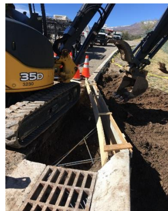
Crew members removed a 6 inch PVC drainage pipe that was plugged and installed a new 12 inch culvert and modified the drop inlet to take more water near the 10th hole T-box at the Golf Course
