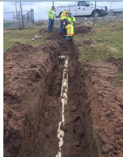
Crew members removed a 6 inch PVC drainage pipe that was plugged and installed a new 12 inch culvert and modified the drop inlet to take more water near the 10th hole T-box at the Golf Course
