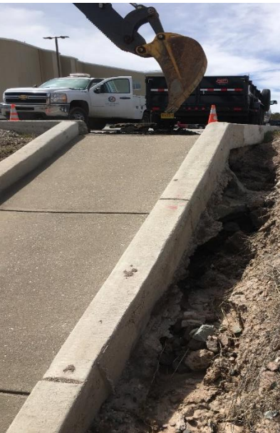
A section of pavement at the Pajarito Cliffs Site collapsed from drainage issues. Staff repaired this section of pavement and fixed any potential for further drainage issues.
