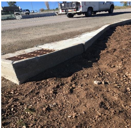
Crew members removed a 6 inch PVC drainage pipe that was plugged and installed a new 12 inch culvert and modified the drop inlet to take more water near the 10th hole T-box at the Golf Course
