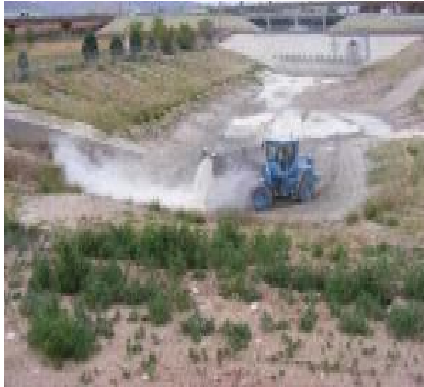
An El Paso Water Utilities employee spreads recycled gypsum at the Saipan Basin stormwater retention pond. The gypsum conditions the clay under the pond to improve water percolation and drainage so that there is less of the standing water mosquitoes need for breeding.
