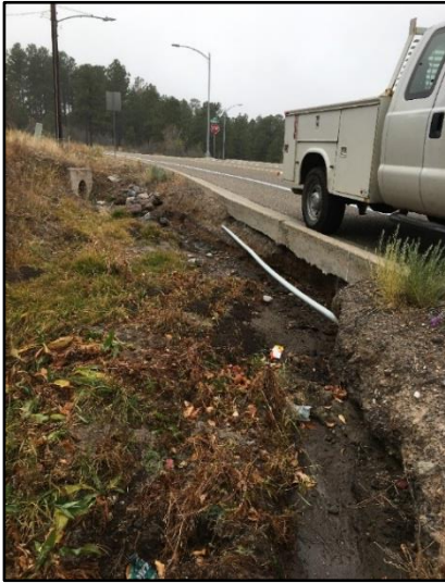
Crews repaired a drainage ditch and covered exposed lines along Canyon Road east of Central Avenue.
