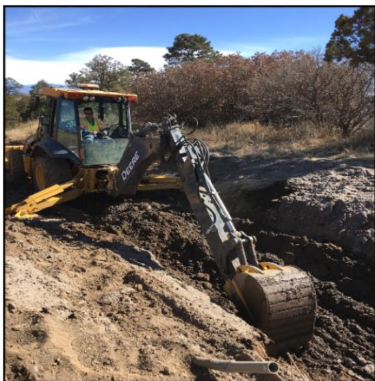
Crews cleared a culvert on North Mesa.
