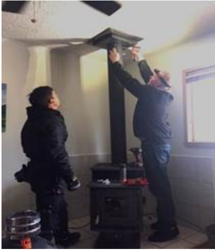
Home Rehabilitation Project (Los Alamos) Wood Stove Flue Replacement
