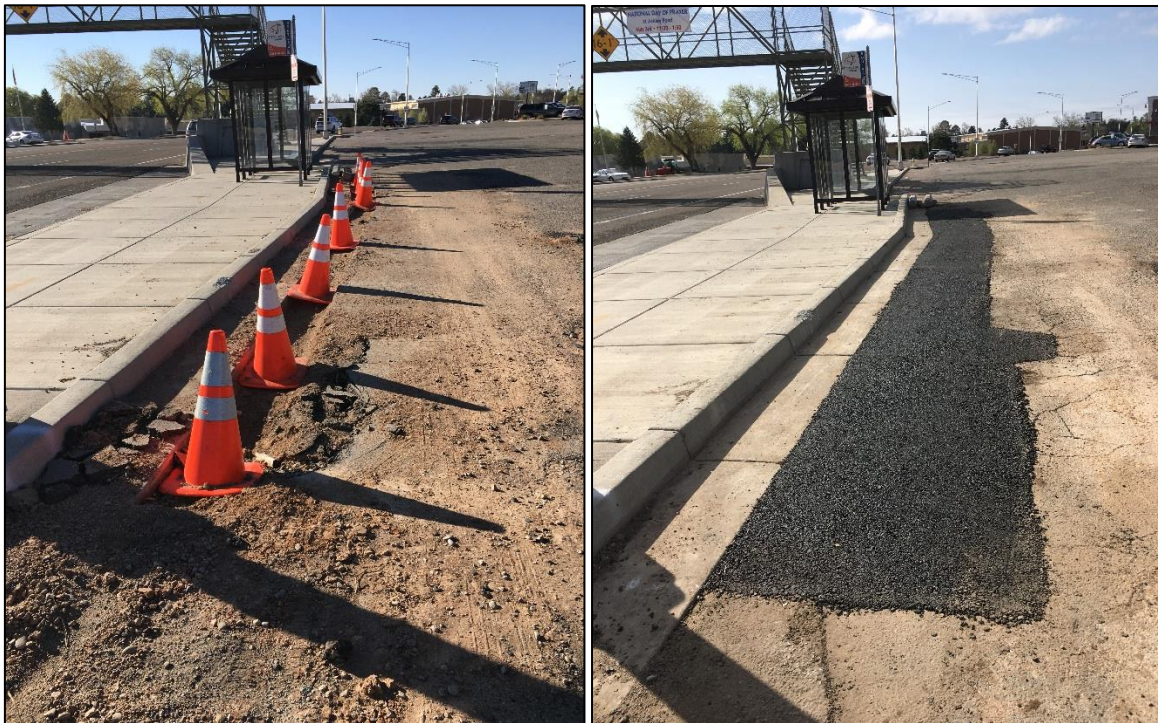
Crews patched a section of road cut by the Utilities Department in the parking lot near the Morning Glory restaurant.
