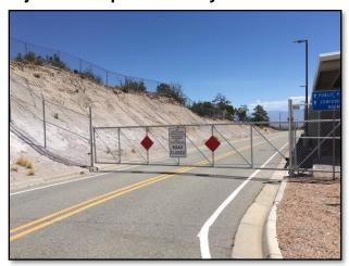
An automated operator has been installed on the new gate designed to better secure PCS buildings #1, #4, and #5 located outside the yard. The gate is now programmed for automated closure to prevent entry during the overnight hours and on weekends. Vehicles needing to exit from within the gate can now do so without the need to stop and unlock the chain previously used to secure the gate after hours.
