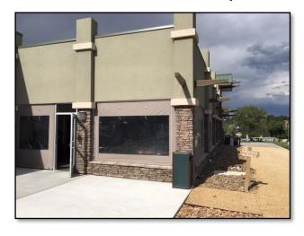
The patio enclosure at Cottonwood on the Greens suffered damage from a burst of extremely high wind such that the pictured exit door was completely blown off the frame and several windows in the canvass siding were stressed to the point of beginning to tear apart. Facilities Division staff worked to purchase the necessary hardware to repair the door and reinforced stitching was done to the canvass around window areas where necessary.
