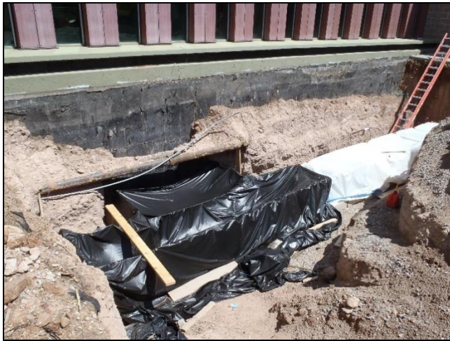
Library air intake excavation and piping
