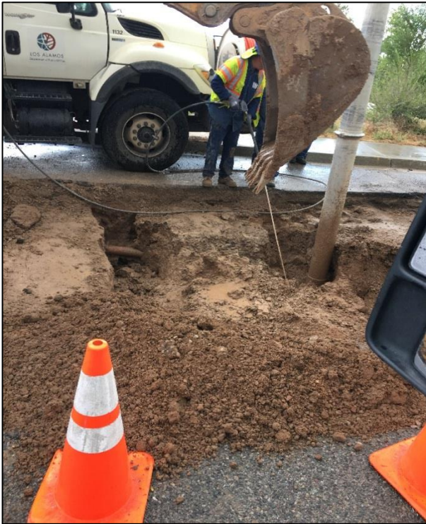
Crews assisted in repairing a patch from a broken water main on Arizona.
