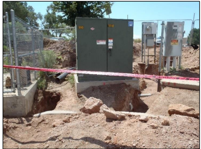
Utility yard trenching for new gas/electric
