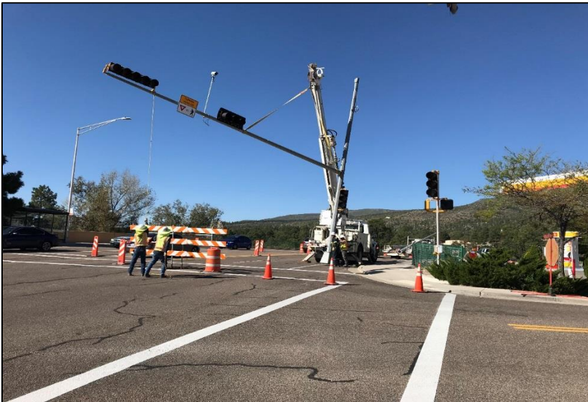
Traffic Electricians assisted and supervised the installation of the traffic signal pole at Diamond Drive and Arkansas. This pole was knocked down in an accident and had to be replaced. Electrical Contractor Bixby Electric was hired to do the installation.
