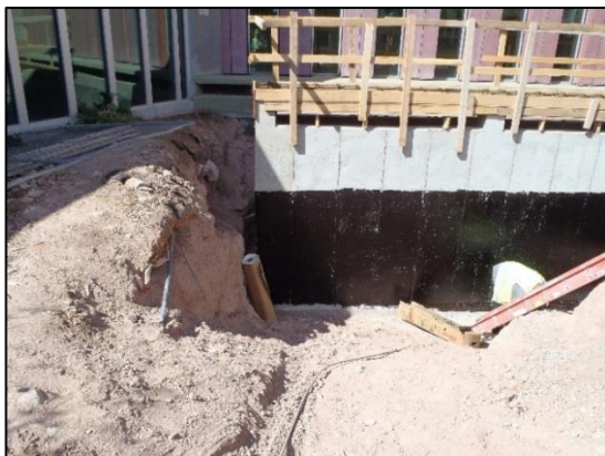
Library Air Intake and Waterproofing
