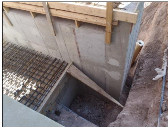
Connection between new and old Intakes
