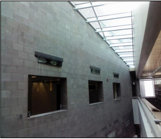
New return air penetration (smaller holes)
