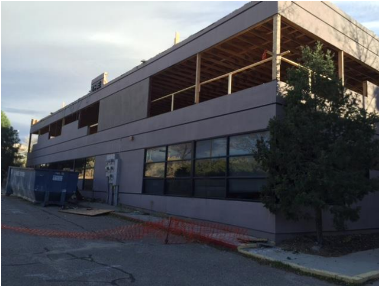
Construction has begun on the third story going up on the Oppenheimer building
