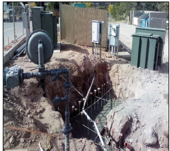
New gas meter and transformer (upper)
