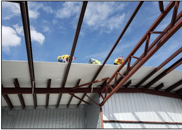
Crews install roofing on the new hanger structure
