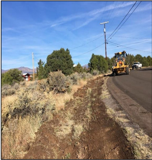
Crews defined a ditch on South Monte Rey where a resident was concerned about storm water flooding her house.
