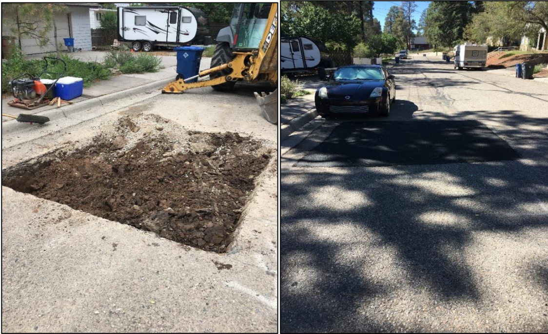
Crew's crew patched a portion of road on 40 th street where GWS had to repair a line.
