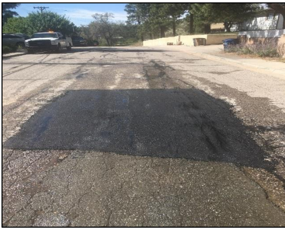
Crews repaired a pot hole on 41 st Street.
