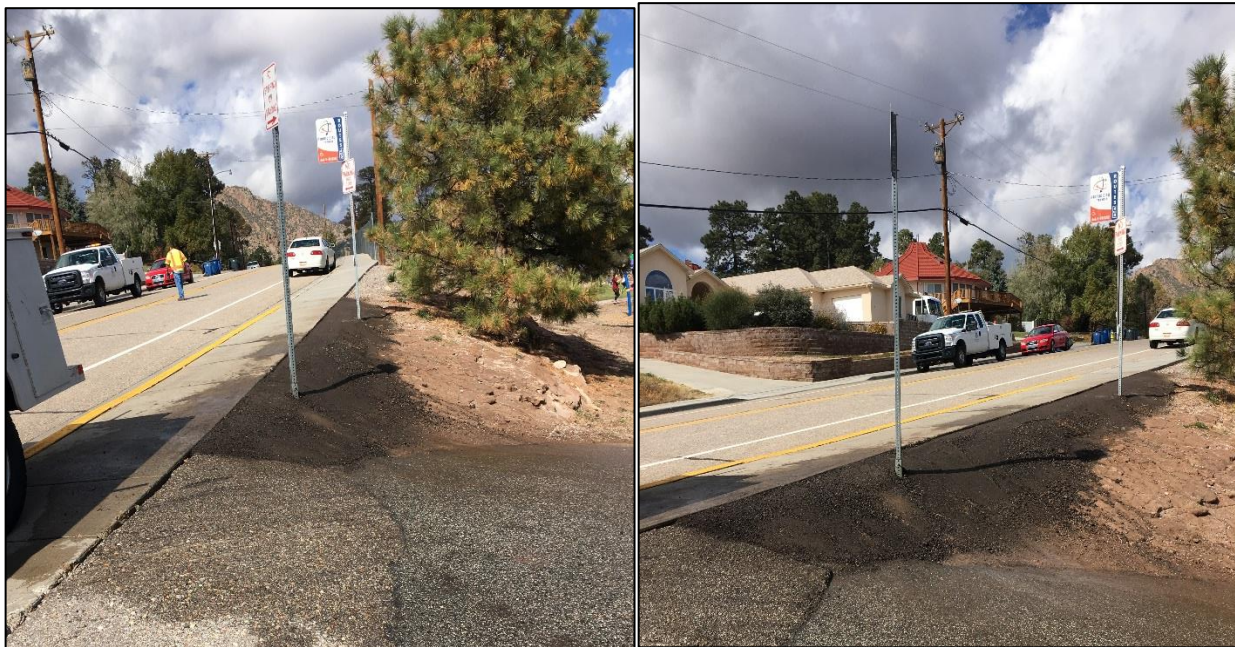
Crews built up a shoulder near Mountain Elementary School where storm water was undermining the curb/gutter and roadway.
