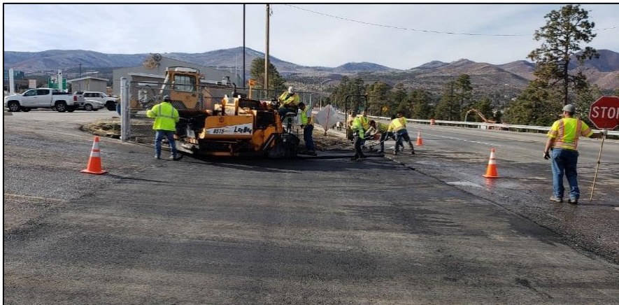
Crews finishing placing asphalt at the Eco station to mitigate water ponding and ice forming in an area where employees walk to open and close the gate.
