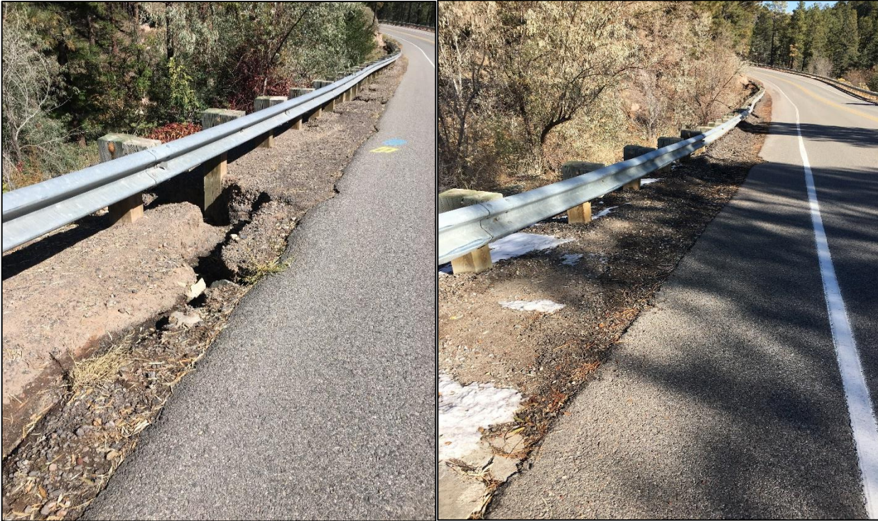
Crews repaired a section of shoulder under an existing guard rail where the soil was eroding from the recent rains on Range Road.
