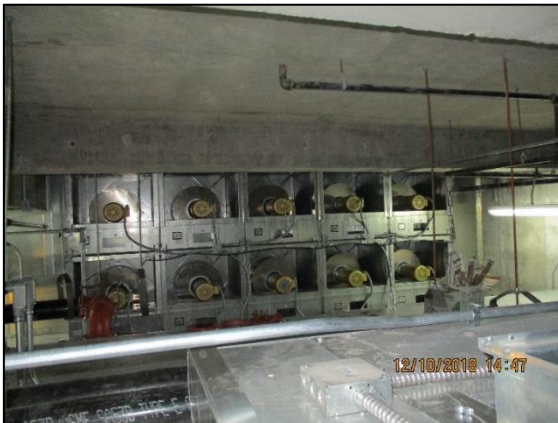
Newly installed fan units.
