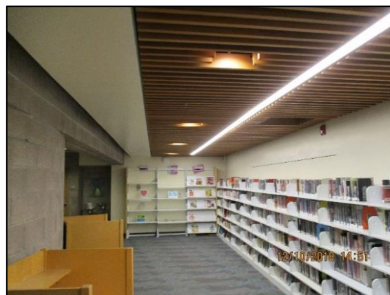
Newly installed wood ceiling and LED lighting in lower level.
