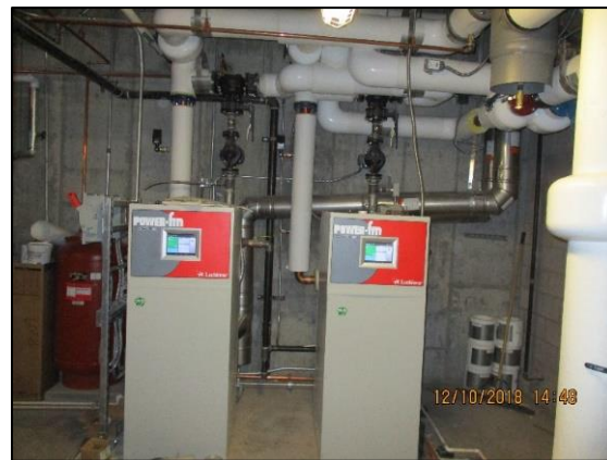
Newly installed boilers.
