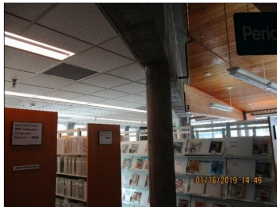
New LED lighting comparison. New (Left), Old (right).
