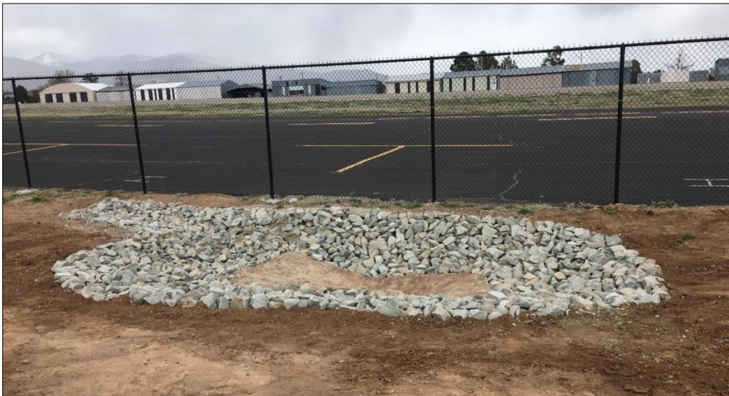
Crews fixed erosion issues and placed rock to prevent future erosion at a drain located on 502 near the airport.
