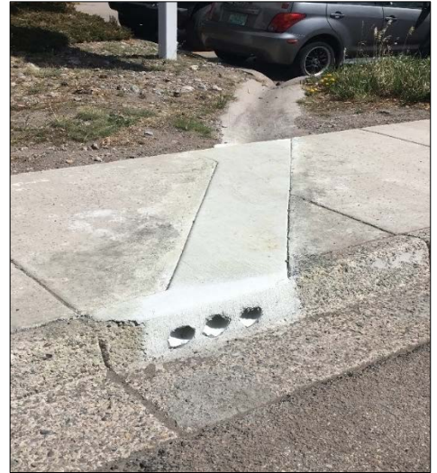
Crews eliminated a metal drain plate which was continual tripping hazard and replaced it with pipe with concrete.
