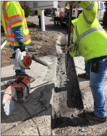
Crews eliminated a metal drain plate which was continual tripping hazard and replaced it with pipe with concrete.
