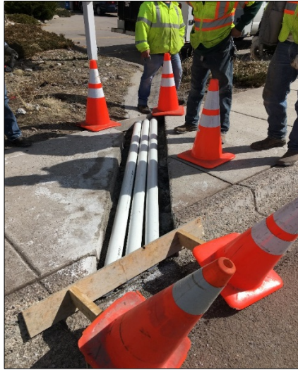
Crews eliminated a metal drain plate which was continual tripping hazard and replaced it with pipe with concrete.
