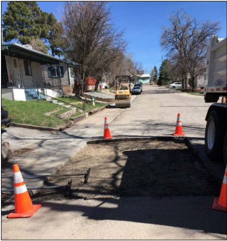
Crews assisted GWS in repairing a patch of asphalt that was removed for a water line repair on 36 th Street
