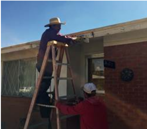
Roof and fascia repair for White Rock home
