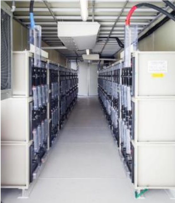
800 kW x 2.3 MWh lead-acid battery
