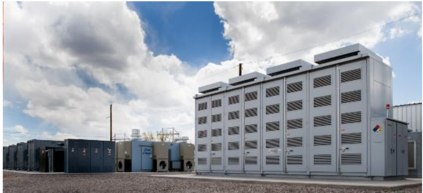
1-MW x 6 MWh NaS battery
