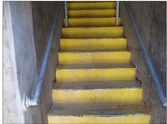
Figure 2 – Deteriorated Steps
