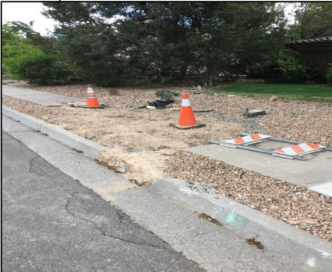
Crews repaired curb and gutter and sidewalk at 718 Jeffrey Pl. due to a water break.
