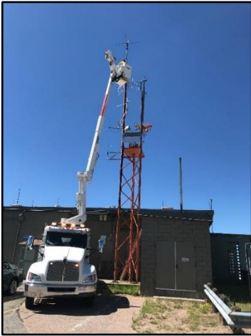
Crews repaired an obstruction light at the Airport.
